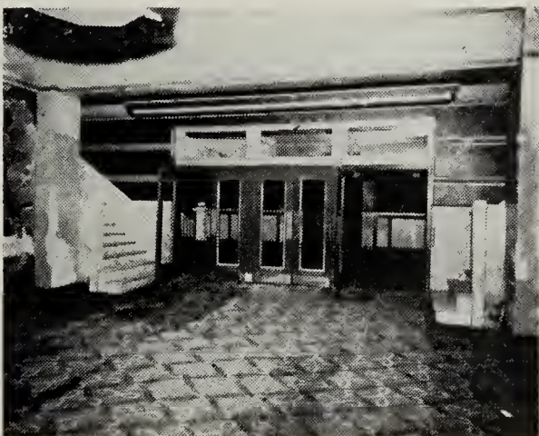
Unightly doors were removed from the old lobby, above, and walls were covered with plaster, and painted turquoise. With terrazzo flooring and clean, functional lines, the lobby has been transformed into the well-planned area seen at right.
